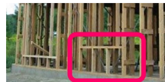
Example of platform construction.
