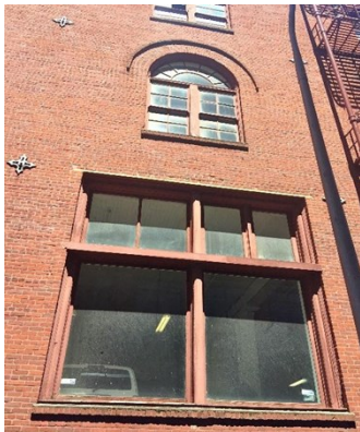
Note tie plates in place as well as the arched spandrel above the upper window. A lintel can be noted above the double windows to provide reinforcement and serve as a small header.
