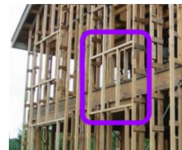
Example of balloon frame construction.
